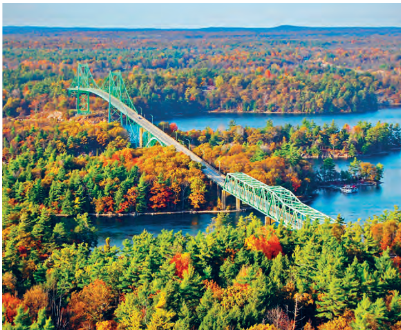
Thousand Islands International Bridge
